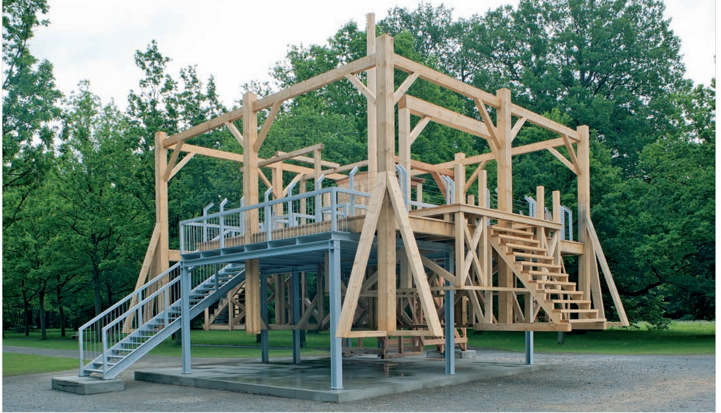
SAM DURANT Scaffold , 2012. Designed by Sebastian Clough with punkt vier architekten and Klute & Klute Ingenieurbüro. Commissioned and produced by dOCUMENTA (13) with the support of Blum & Poe, Sadie Coles HQ, Paula Cooper Gallery, Praz-Delavallade. Foto: Nils Klinger. Cortesia: Sam Durant; , Blum & Poe, Sadie Coles HQ, Paula Cooper Gallery, Praz-Delavallade.
